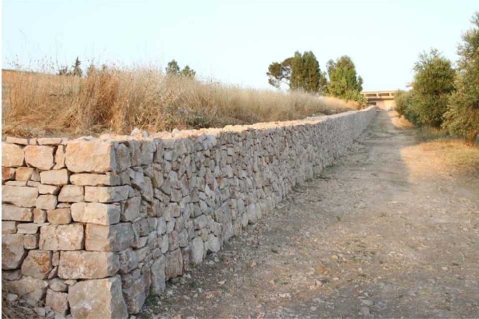
Figure 2 - Dry-stone wall constructed under the ARUPA Project.
