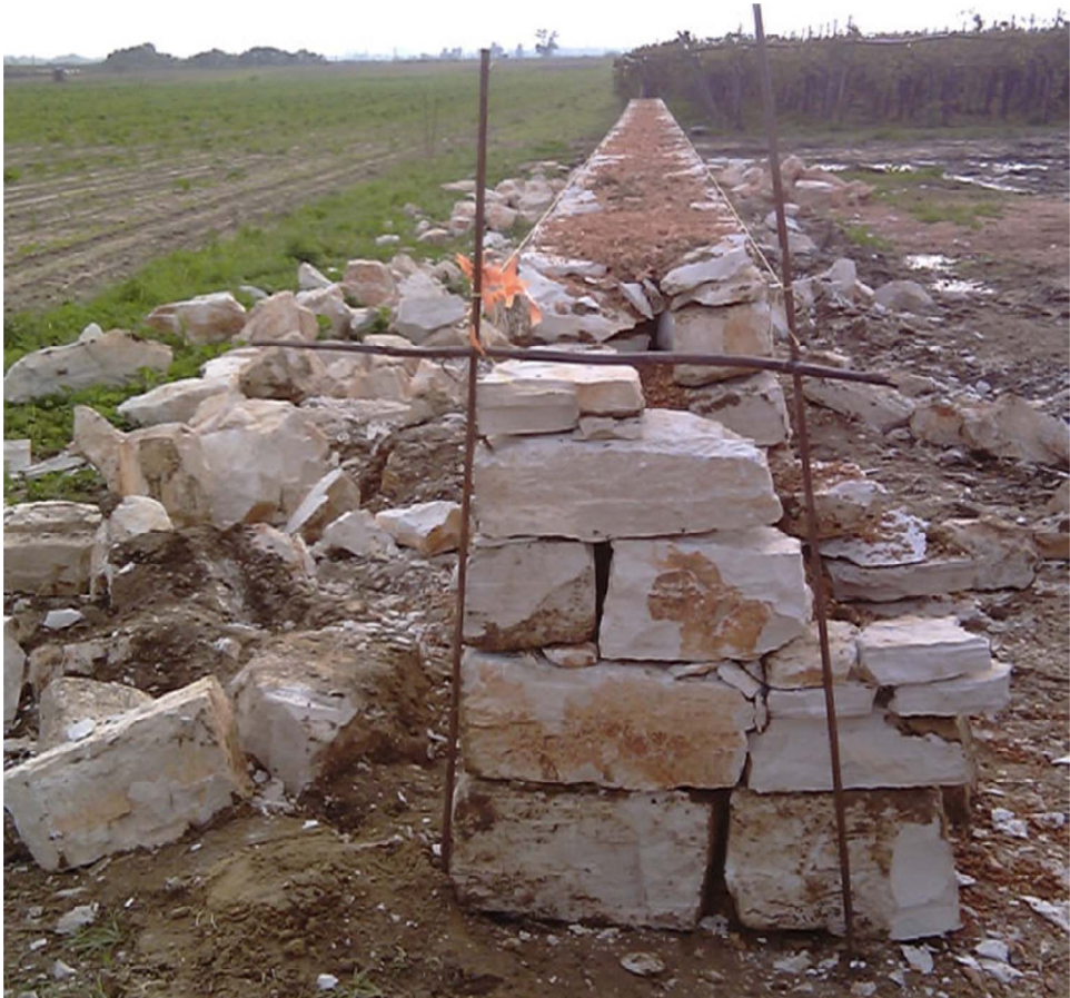
Figure 1 - Construction of a new dry-stone wall under the ARUPA Project.
