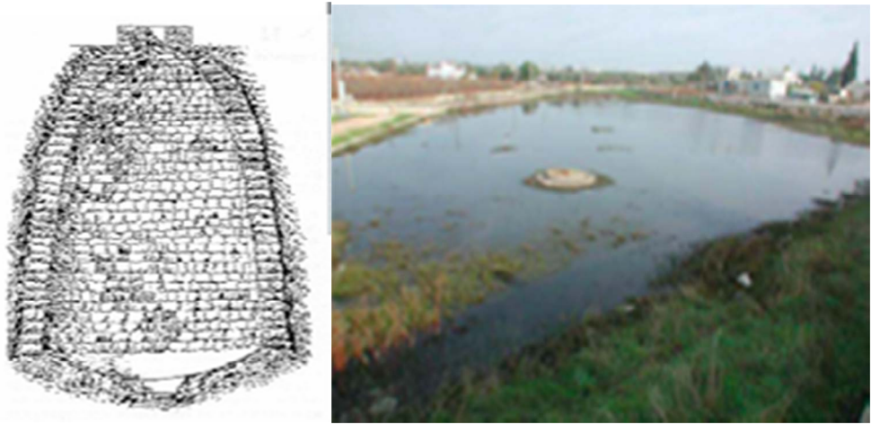
Figure 4 – Scheme of a traditional grounded water storage tank (a); Grounded water storage tank/vernal pool realized under the ARUPA Project (b).
