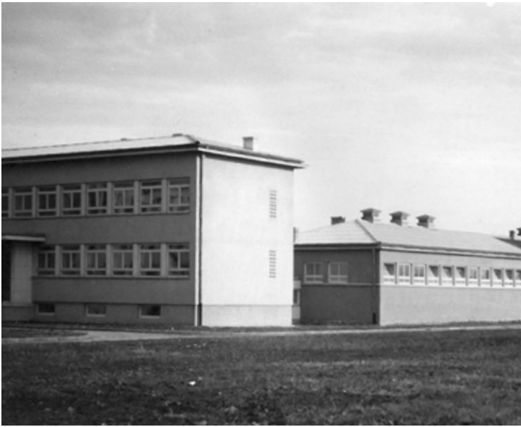
Detail of the completion of the construction of the Clinical building of the Faculty with the adaptation of the access road in 1959 (Faculty Archives).
