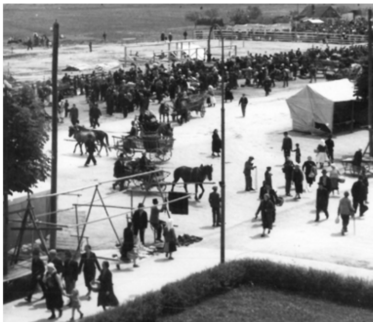
The fair on Heinzlova Street in 1938. In the background is the construction site of the Faculty of Veterinary Medicine (Faculty Archives).
