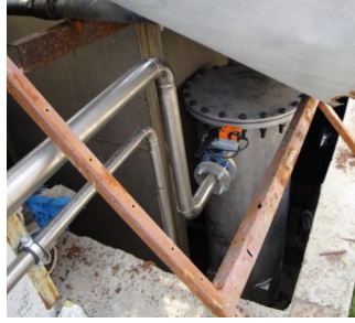
Figure 1. Pressurized capsule within the DAF circuit
