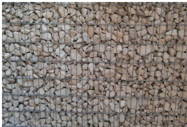
Figure 6. Side stone wall
