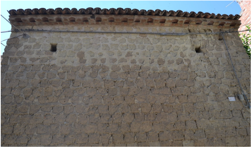
Figure 1. Earthen vernacular rural building in Basilicata Region.
