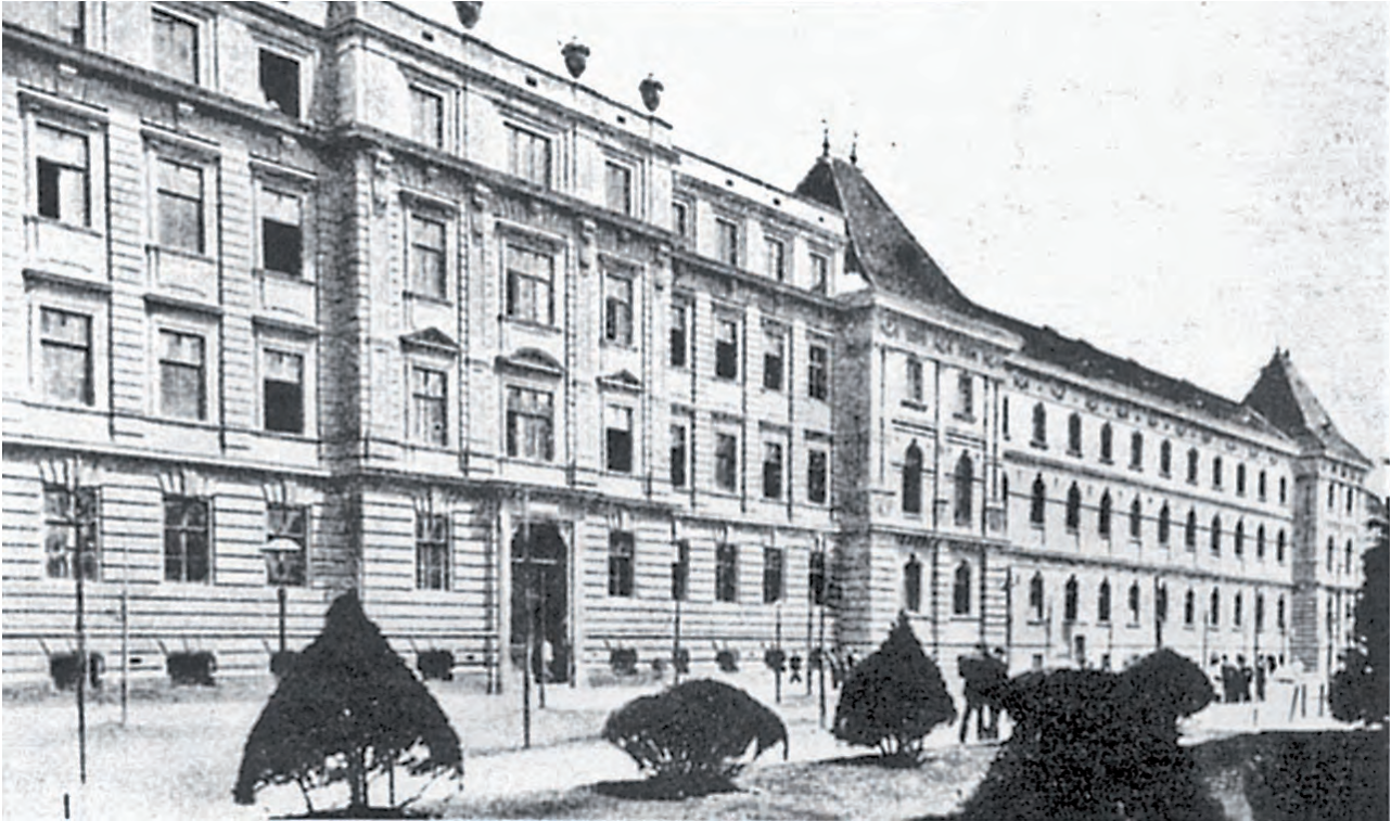
The first building of the Technical College
