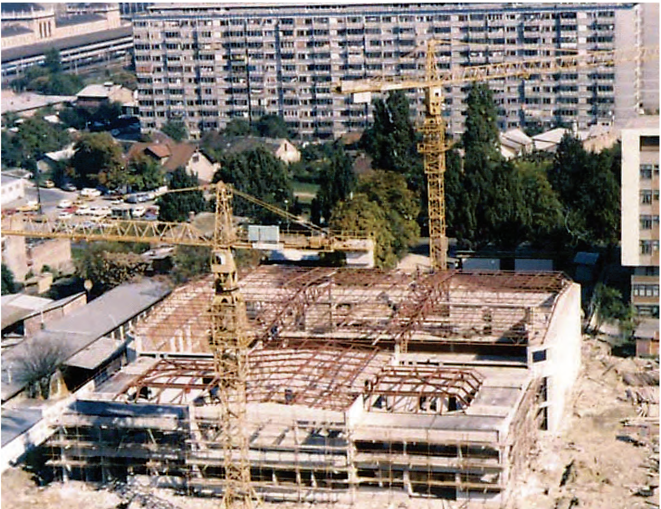
Construction of Martinovka Sports Hall.
