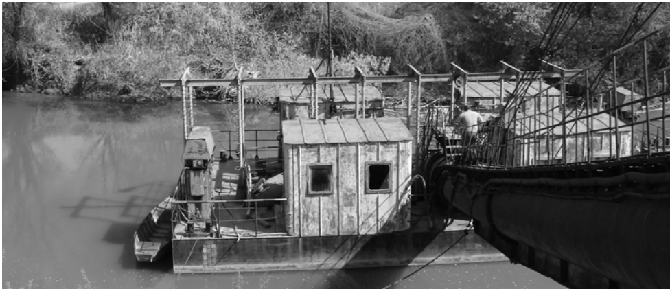
Figure 6 Ship of Floating Pumping Station on Mures River [2]
