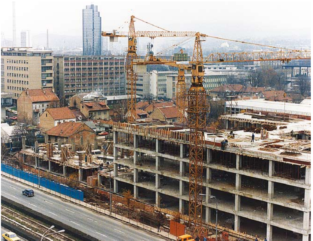
Construction of the Faculty's "D"-building in late 80-ies.
